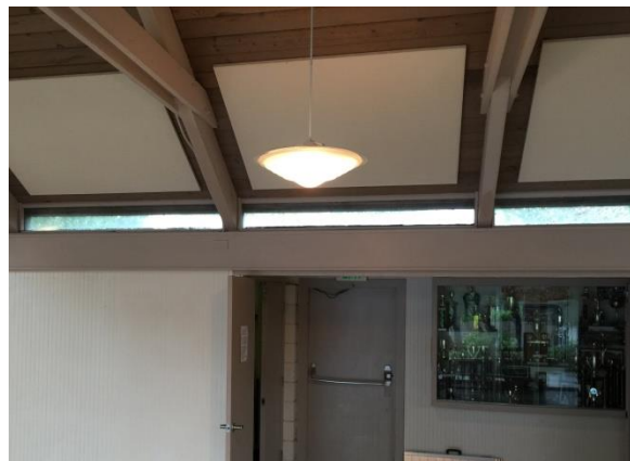
Fig. 5, Clear Story Windows
